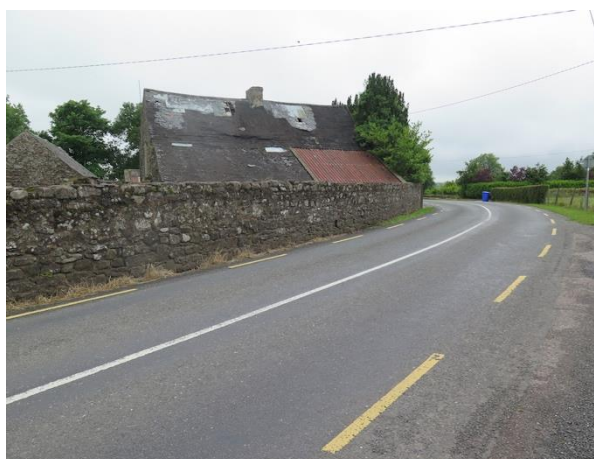
Figure 15-46: Western TDR area at Ballynoony West, facing southwest
