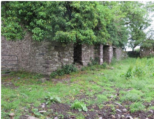
Figure 15-39: Building at Castlebanny deserted farmstead
