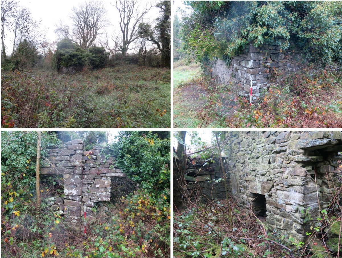
Figure 15-24: Views of ruined building directly north of T21 location
