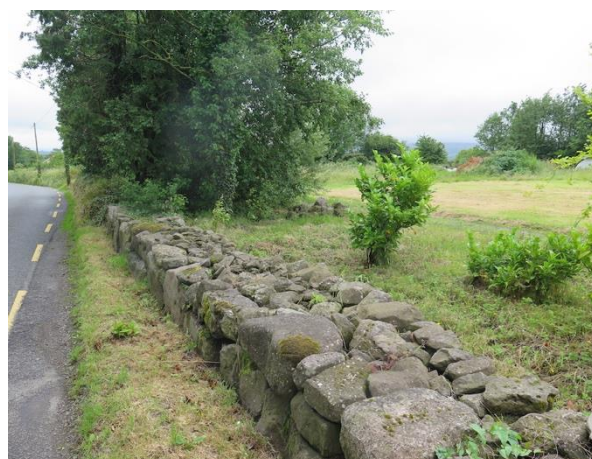
Figure 15-47: Western TDR area at Ballynoony West, facing south
