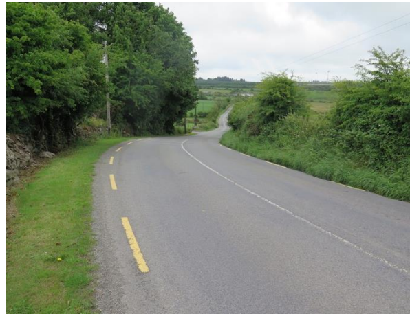
Figure 15-50: Eastern TDR area at Ballynoony West, facing east
