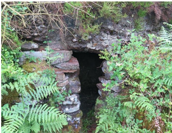
Figure 15-33: Entrance to structure KK036-040
